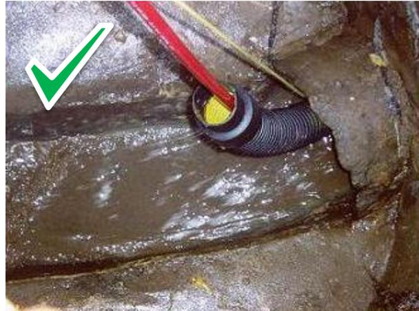
*A typical guide that can avoid contact between the hose and any sharp edges in the sewer.*
